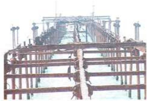
Fig 3.1 Existing pier structure in Alappuzha
